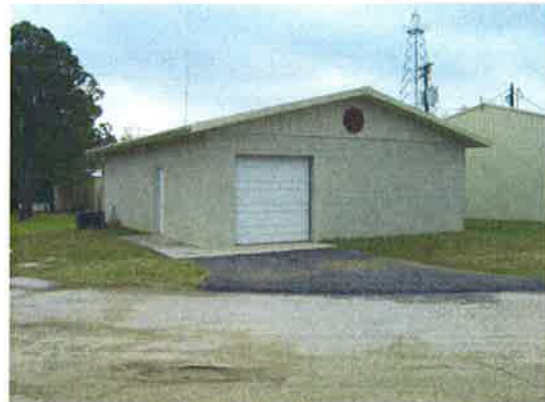
New Records Storage Facility
